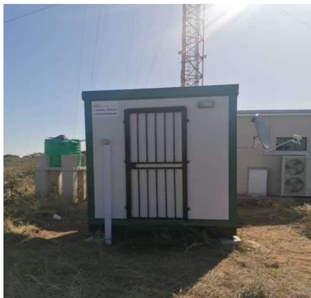
Figure 29: Shelter housing the Integrated FM at Senyamadi Transmitter System
