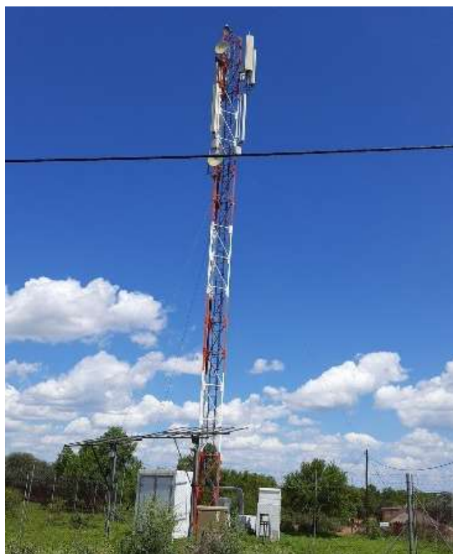
Fig. 41: A Typical Base station
