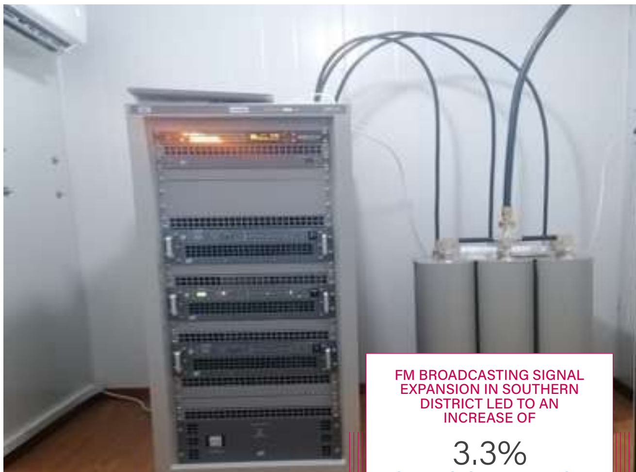
Figure 28: Integrated FM Transmitter System
