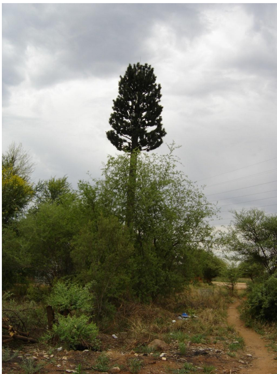
Figure 9: A Base Station Tower that matches the surrounding environment
